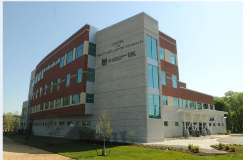
Pictured: The Center for Health Education and Research (CHER) Building in Morehead, KY
